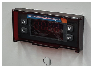
Figure 6: Push controller into the hole. Silicone will seal against mounting surface.
